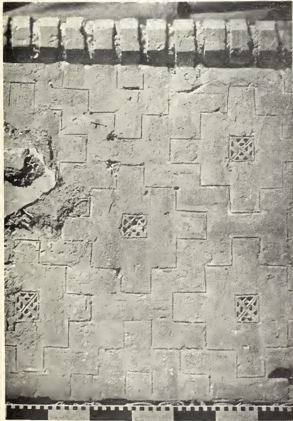
PHOTO. M. B. SMITH, NEG. L-93.35 FIG. 40—SANCTUARY, WALL TO RIGHT OF MIHRĀB, GAÇ POINTING
